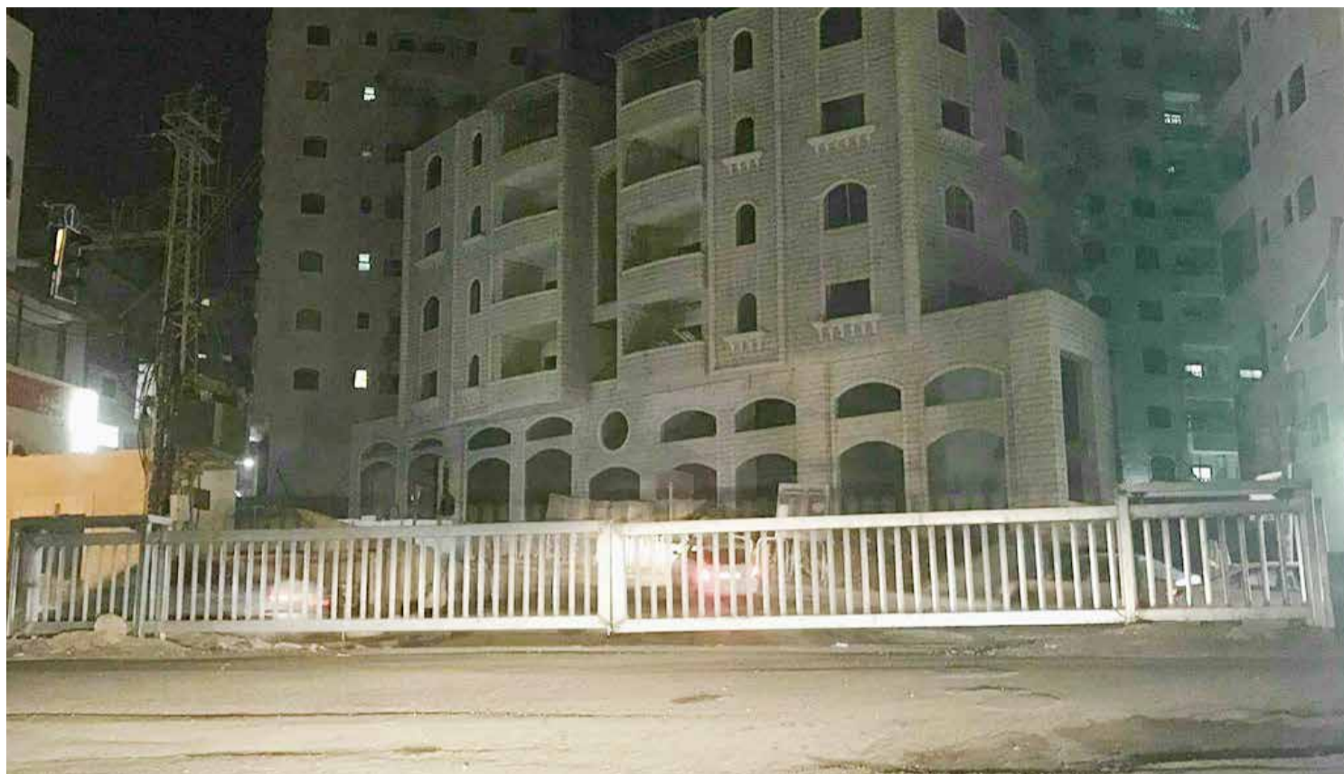
Part of the work for the construction of the gate.
